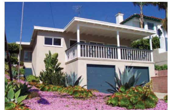
Original home: The Fortunato's original 1959 "post and beam" California home.
